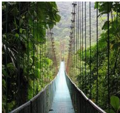
Mistico Hanging Bridges
